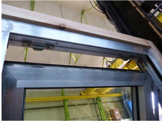
Figure 4 Friction stays and security claws on top hung sash
