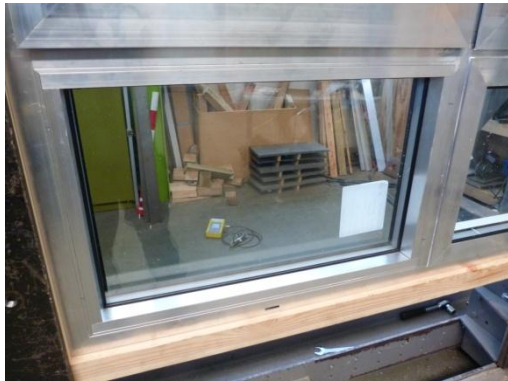
Figure 8 Externally glazed light viewed from attack side
