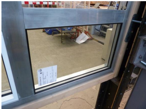
Figure 10 Externally glazed light viewed from non-attack side
