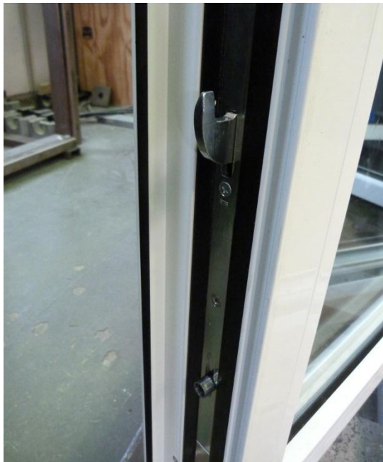
Figure 3 View of lower hook bolt and cam
